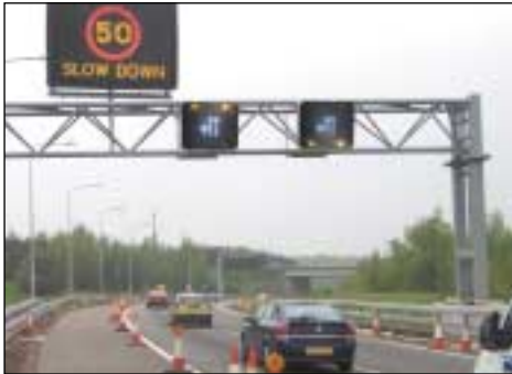
Trial of M42 ATM Active Traffic Management Scheme
